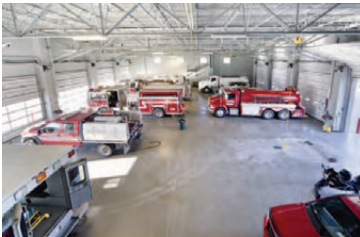
Today's larger fire apparatus require taller and wider bay doors, along with the increased aisle space and cab-tipping height in the apparatus room.
